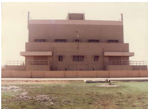
Figure 2: Sludge Hygienisation Research Irradiator (SHRI) Facility, Baroda
